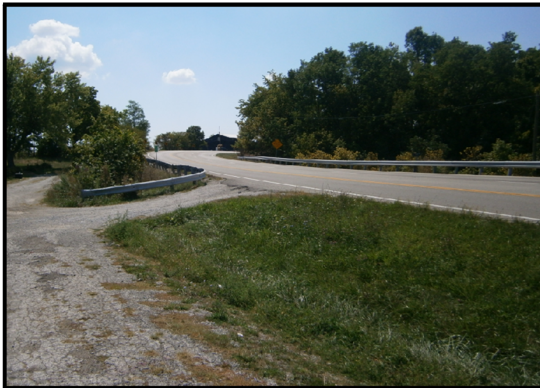
Exhibit 2: Southern Curve at MP 12.0 Looking South
